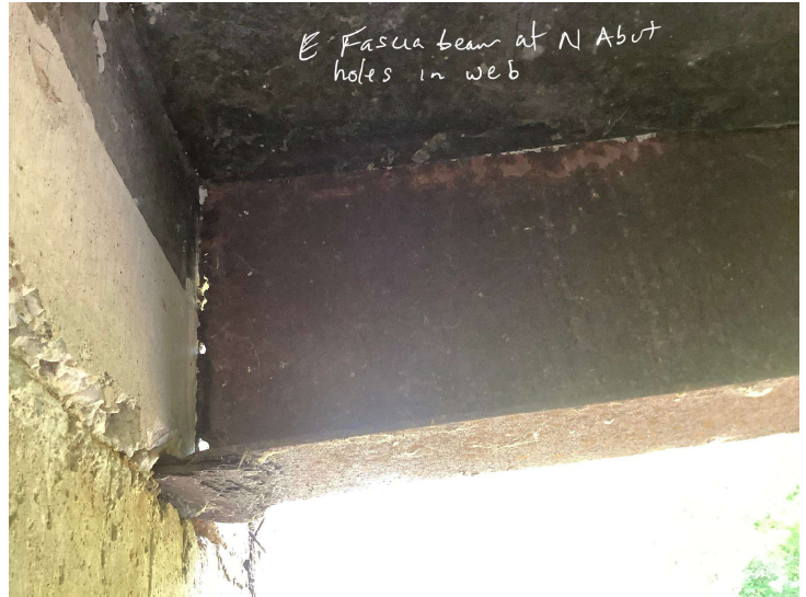
Document Name: IMG_3421.JPEG Category: Superstructure Span Number: Comments: East fascia beam at north abutment, holes in web
