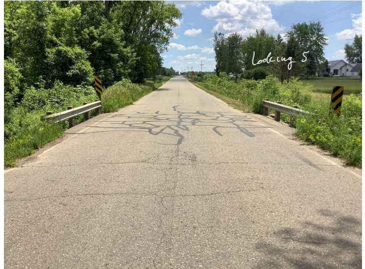
Document Name: IMG_3374.JPEG Category: Approach Span Number: Comments: Looking south
