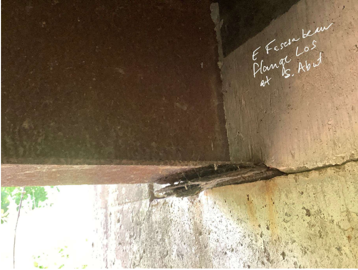
Document Name: IMG_3401.JPEG Category: Superstructure Span Number: Comments: East fascia beam, flange LOS at south abutment
