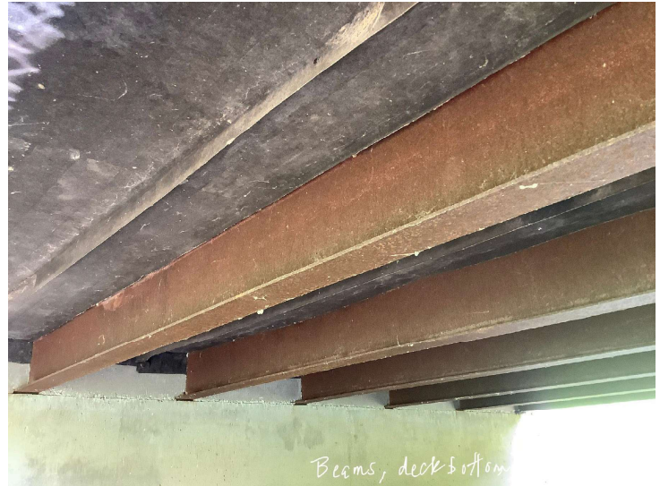
Document Name: IMG_3398.JPEG Category: Superstructure Span Number: Comments: Beams, deck bottom
