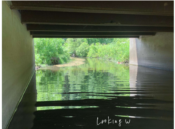
Document Name: IMG_3405.JPEG Category: Channel Span Number: Comments: Looking west
