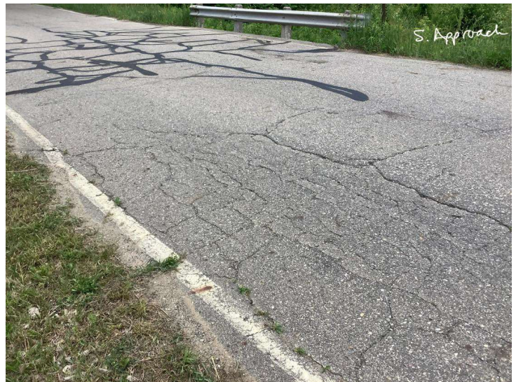
Document Name: IMG_3389.JPEG Category: Approach Span Number: Comments: South approach
