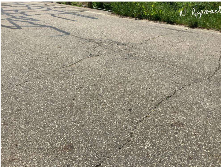
Document Name: IMG_3378.JPEG Category: Approach Span Number: Comments: North approach
