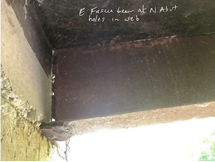
Document Name: E Fascia at N Abut (1).jpg Category: Superstructure Span Number: Comments: East Fascia Beam, North End, Holes in Web
