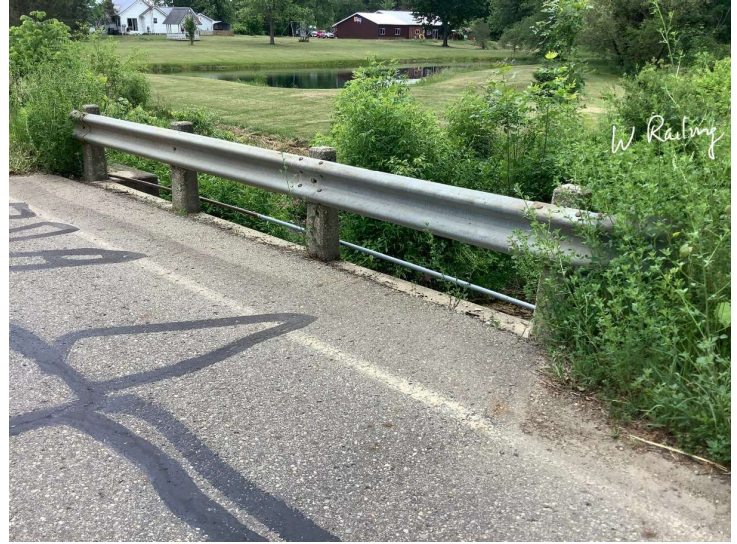
Document Name: IMG_3381.JPEG Category: Railing Span Number: Comments: West railing
