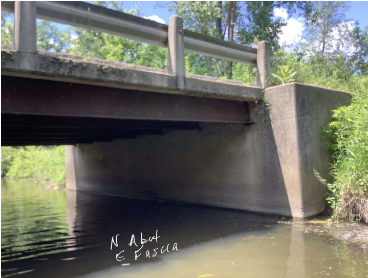
Document Name: IMG_3406.JPEG Category: Substructure Span Number: Comments: North abutment, east fascia
