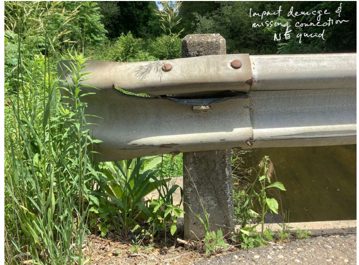
Document Name: IMG_3384.JPEG Category: Railing Span Number: Comments: Impact damage and missing connection, NE quad
