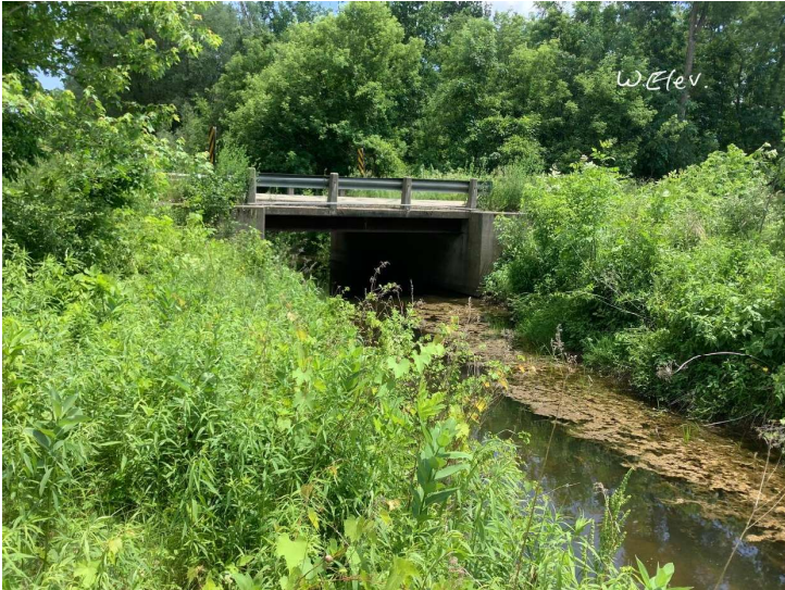
Document Name: IMG_3372.JPEG Category: Elevation Span Number: Comments: West elevation
