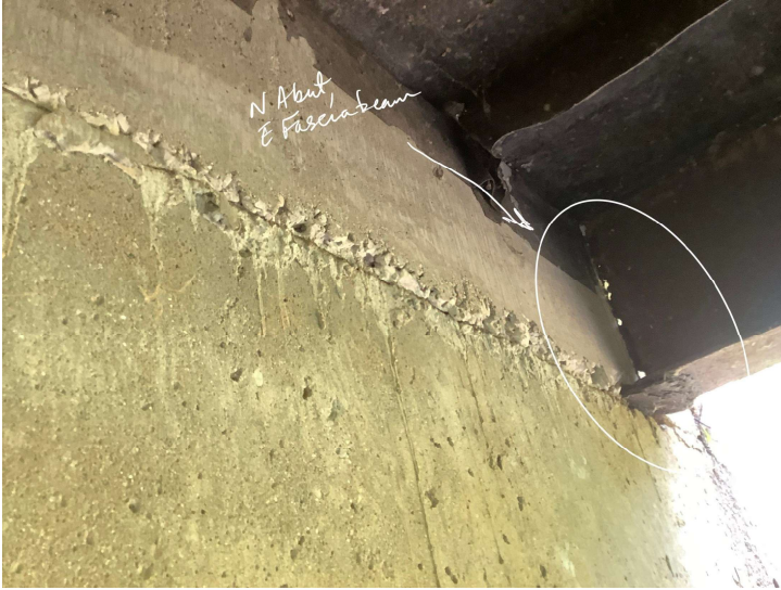
Document Name: IMG_3422.JPEG Category: Superstructure Span Number: Comments: East fascia beam at north abutment, holes in web
