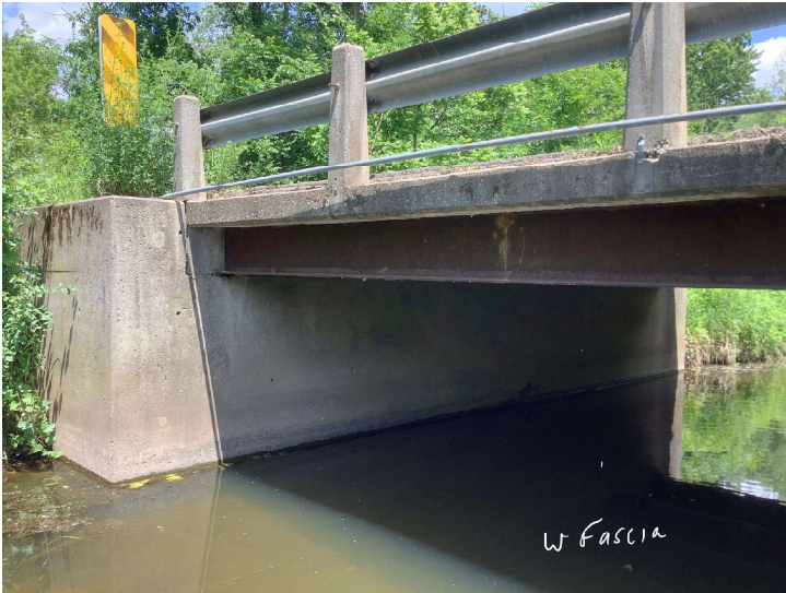
Document Name: IMG_3395.JPEG Category: Superstructure Span Number: Comments: West fascia
