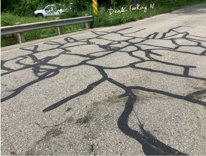
Document Name: IMG_3387.JPEG Category: Deck Span Number: Comments: Deck, looking north
