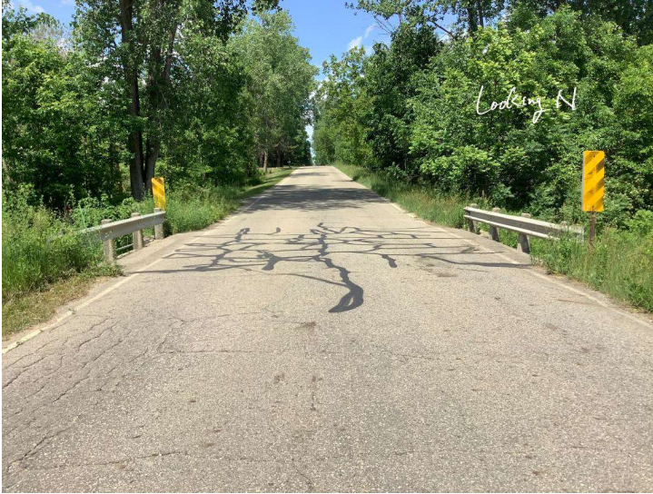
Document Name: IMG_3426.JPEG Category: Approach Span Number: Comments: Looking north
