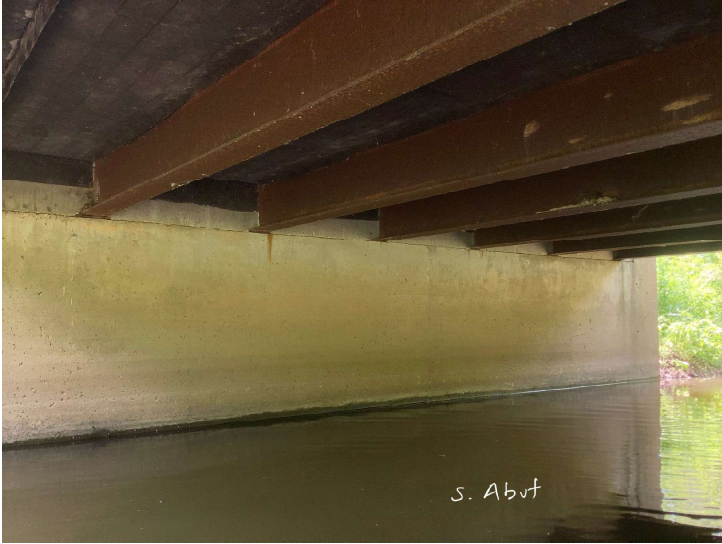
Document Name: IMG_3420.JPEG Category: Substructure Span Number: Comments: South abutment
