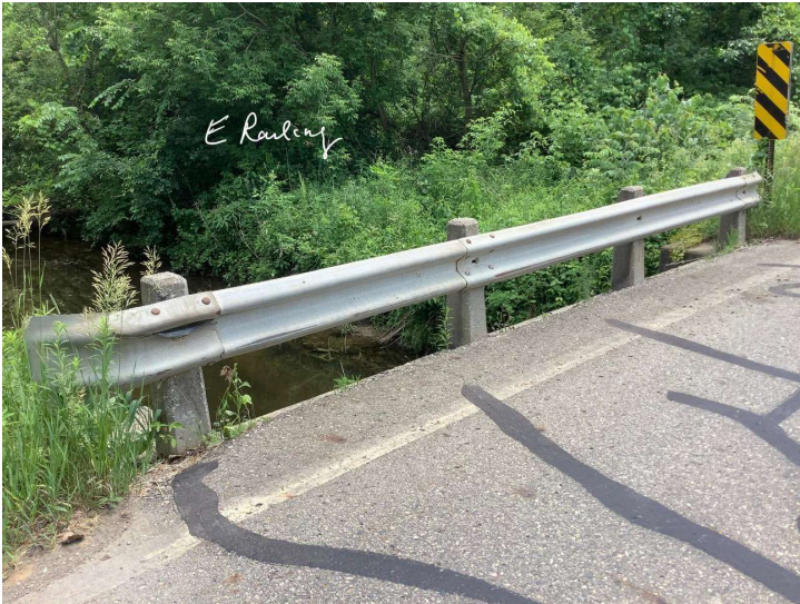
Document Name: IMG_3383.JPEG Category: Railing Span Number: Comments: East railing
