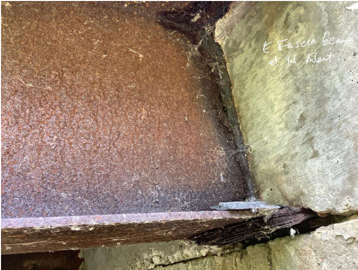
Document Name: IMG_3418.JPEG Category: Superstructure Span Number: Comments: East fascia beam at north abutment
