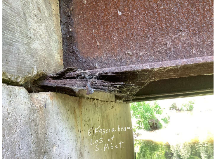
Document Name: IMG_3404.JPEG Category: Superstructure Span Number: Comments: East fascia beam, LOS at south abutment
