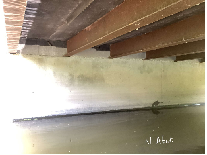
Document Name: IMG_3397.JPEG Category: Substructure Span Number: Comments: North abutment
