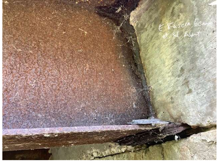
Document Name: E Fascia at N Abut (2).jpg Category: Superstructure Span Number: 1 Comments: East Fascia Beam, North End
