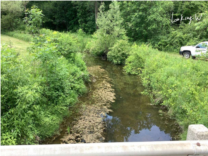
Document Name: IMG_3380.JPEG Category: Channel Span Number: Comments: Looking west
